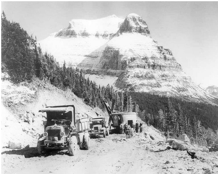
Going-to-the-Sun Road in Glacier National Park, under construction in 1932
