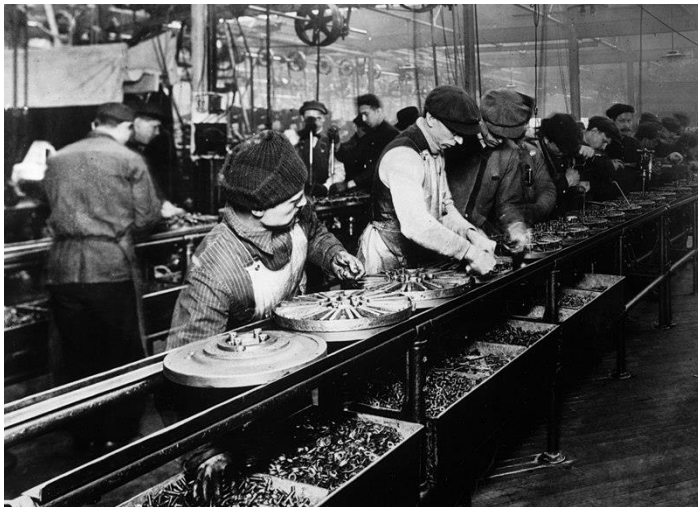
Workers on the first moving assembly line put together magnetos and flywheels for 1913 Ford autos, Highland Park, Michigan, 1913
